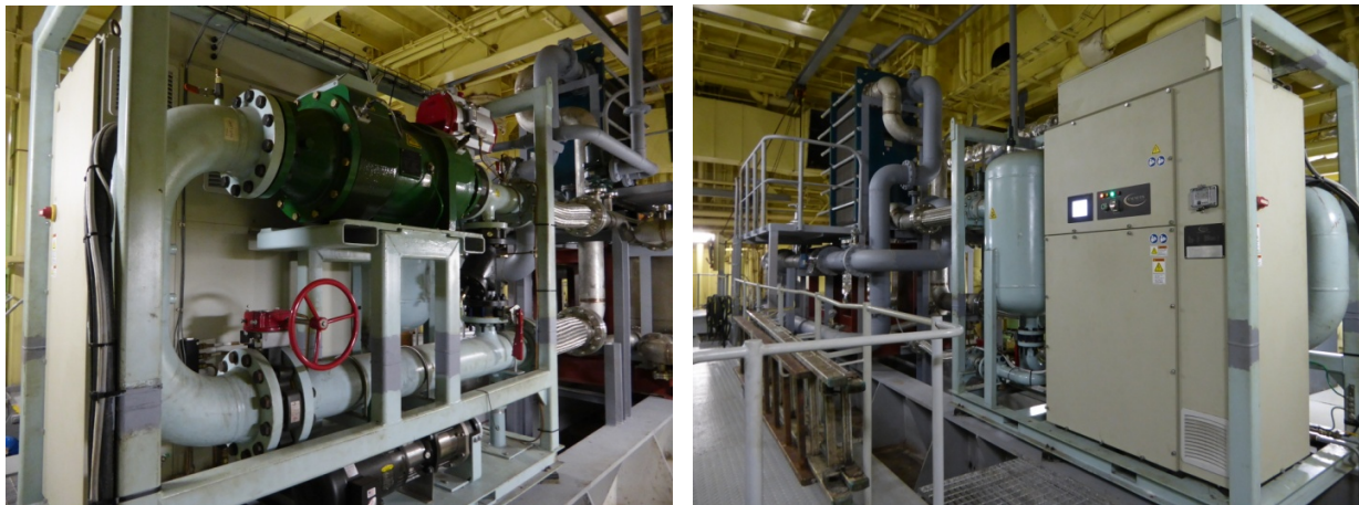
Fig 4-5. Hydrocurrent installation on M/V Arnold Maersk.
